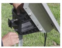
We recommend lining the bracket up with the top of the steel post, once it is in the right position, tighten the U bolts until secure.
