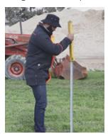
3. Slot the bracket over the post and through the U bolts.
