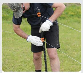
Snap the fence wires to the post using the Insulated Line Post Clip.
