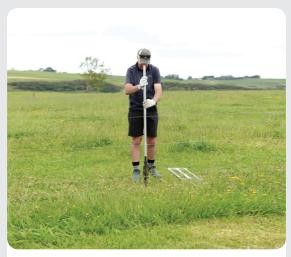
Line up the post to the guide wires. Ensure the wider wings on the foot are running parallel to the fence wire.
