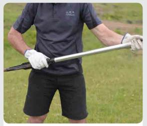
Put sleeve over the post to prevent the post flexing while it is being rammed in to the ground.
