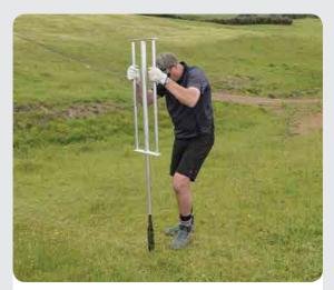
Ram the post in to the ground until the flange on top of the foot is level with the ground.
