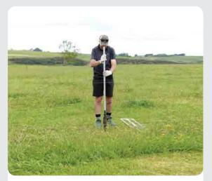
2 Line up the post to the guide wires. Ensure the wider wings on the foot are running parallel to the fence wire.
