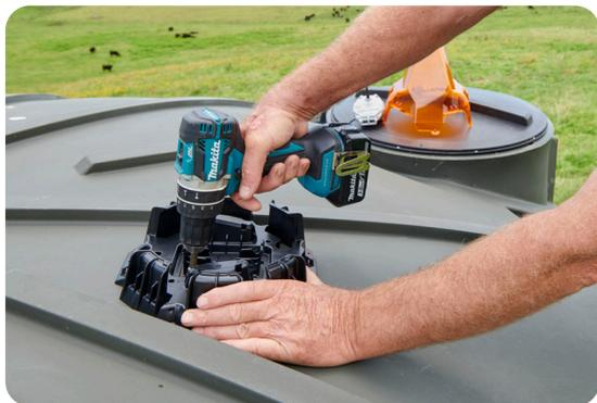
Drill a hole for the sensor cable while being careful to position it above the overflow level. Ensure the hole is smooth so it won't damage the cable.
